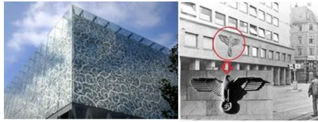
Figure 5. (a)John Lewis Department Store, Leicester, England; (b) Nazi eagle on the wall as decoration, Oslo
