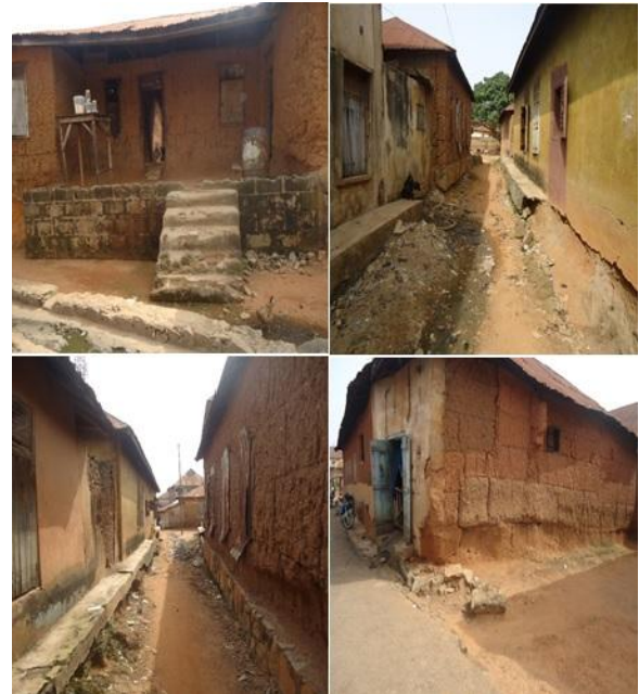
Figure 2: Traditional houses constructed with mud and provided with small sized windows without enough airspaces
